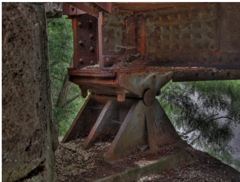
Figure 14.0 “Rust.” These support beams on a bridge are obviously rusted. If the rusting becomes too bad, it will compromise the integrity of the bridge, requiring replacement.
