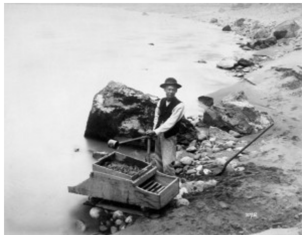
Figure 13.31 Chinese miners introduced machinery like this “rocker” on the Fraser River c. 1875.
