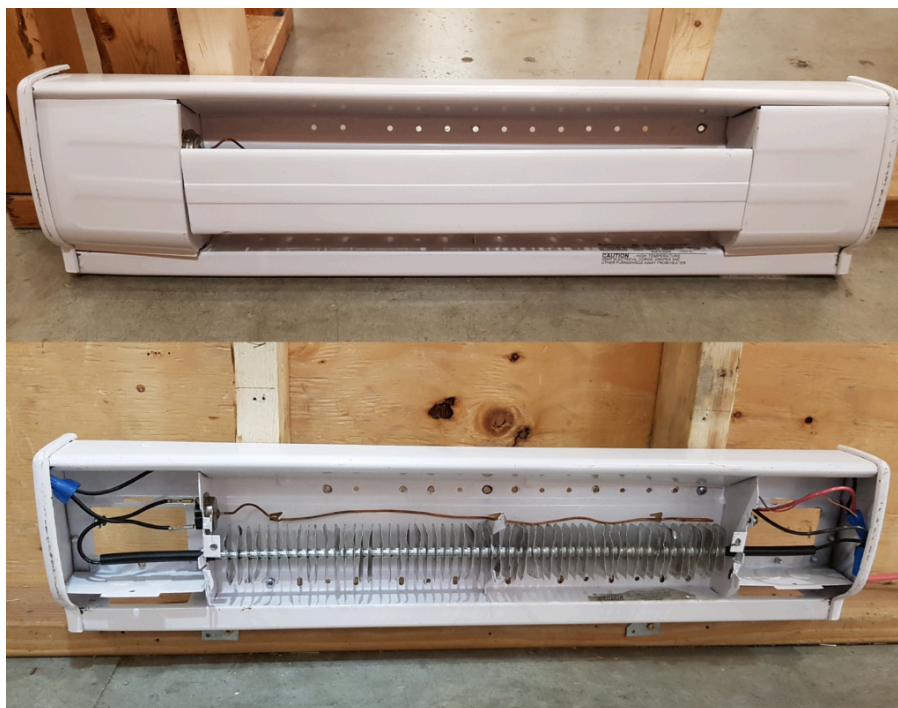
An example of a baseboard heater, both with the cover on, and with the heat fins and wiring connections exposed.
